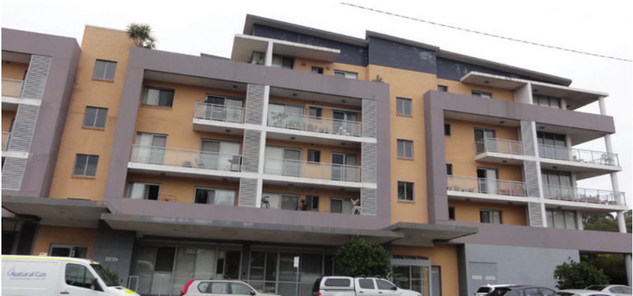
5-Storey residential building on Slade Road
